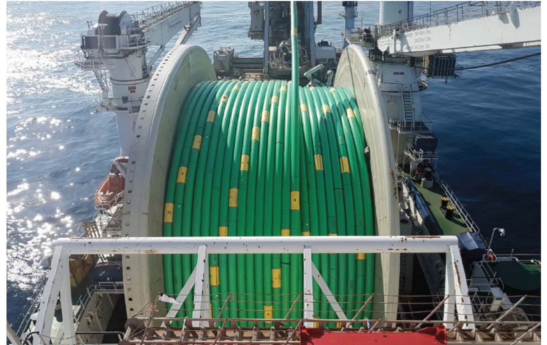
Seven Oceans installing mechanically lined Bubi® pipeline
